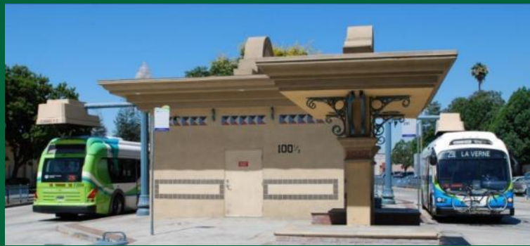
Figure 15: Pantograph chargers at the Pomona Transit Center.
