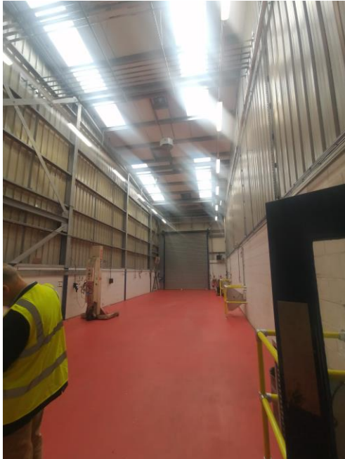
Figure 7: First Bus Hydrogen Maintenance Bay in Aberdeen (UK)
