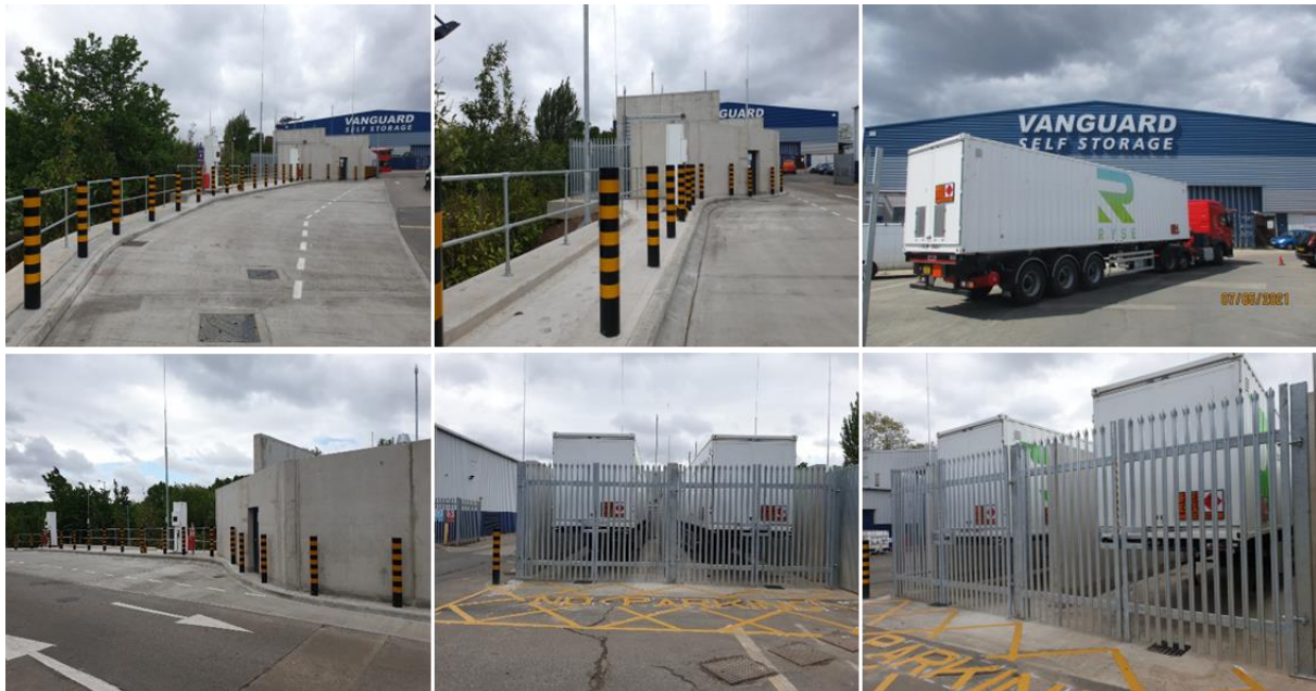
Figure 14: Bus HRS at the Perivale depot and hydrogen transportation to HRS, London
