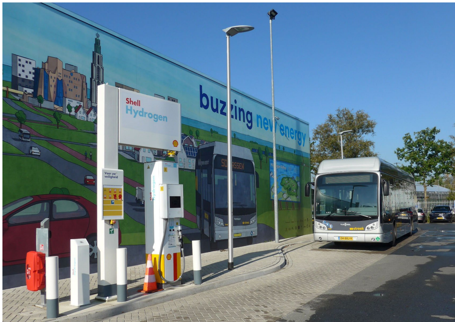
Figure 4-7: Hydrogen dispenser at Peizerweg Depot Groningen, The Netherlands.
