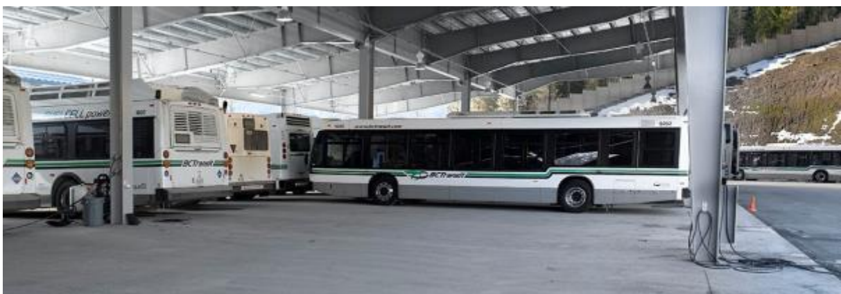
Figure 4: Examples of power outlets at overnight parking
