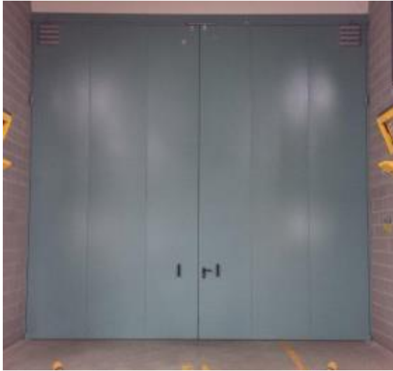
Figure 2: Example of a fire protective door
