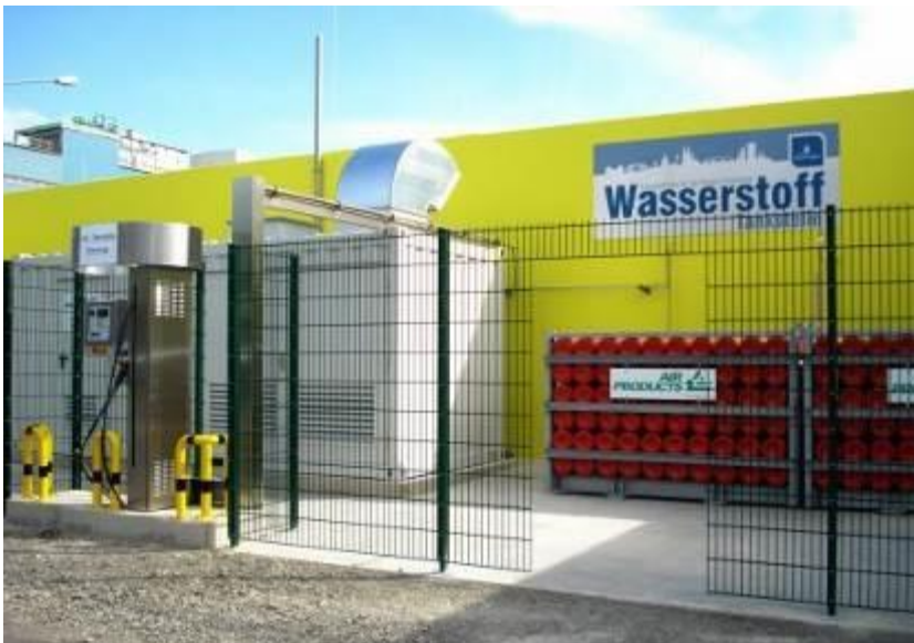
Figure 17: Cologne filling station
