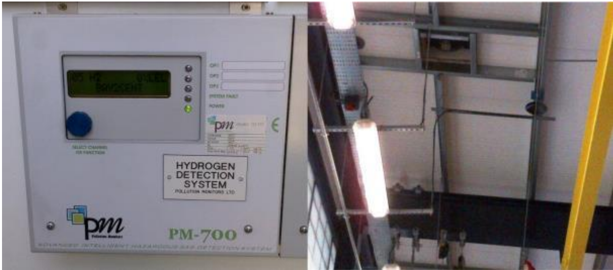
Figure 1: Example of H 2 detection system, H 2 sensors, ventilation and ATEX lights
